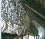
Kitchen oil and grease build-up starts in the metal filters then travels through the hoods and ducts all the way to the roof. It's an ongoing problem that needs a easy cost effective solution.
